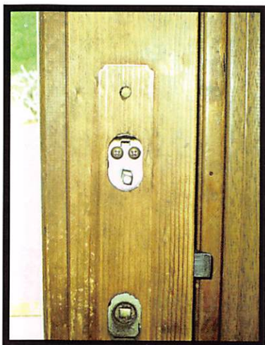
Andersen door with the interior trim removed.
